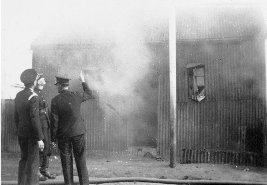
Fig. 2 “The Green House”, an example of a wood-and-iron building in Korsten, Porth Elizabeth, 1938.
