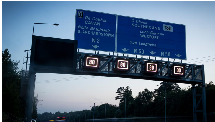
Figure 4.1: Speed advisory system on M50 highway traffic network in Dublin city. Optimal speeds are advised and shown on the screen for each lane on the highway traffic network 1 .
