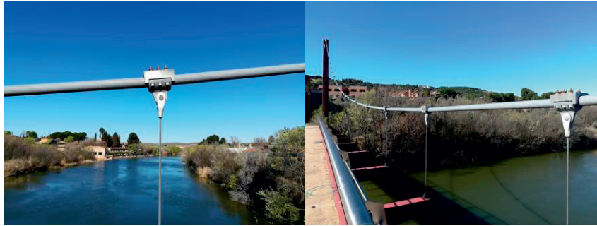
Figure 1: Main cable, hangers and support plates (Polvorines bridge, Toledo, Spain).
