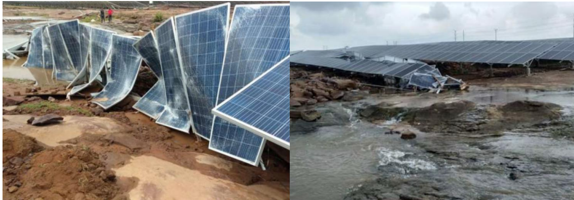
Heavy rains damage solar panels in Madhya Pradesh in 2019 (Source: Marcom India)
