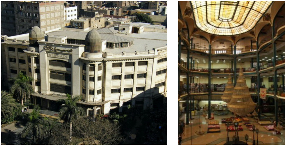
Figure 1. Sednaoui El-khazendar from outside showing main entrance (left) and from inside showing entrance hall, upper floors and central skylight (right).
