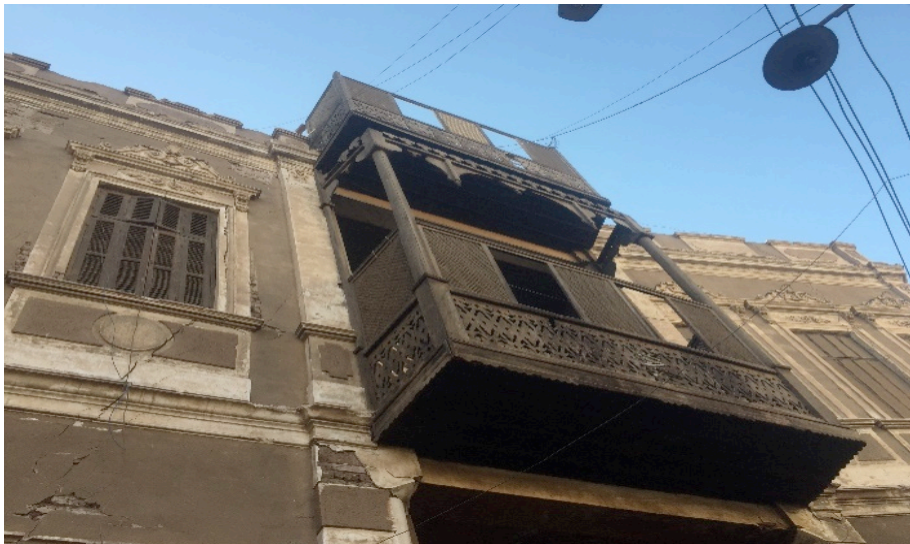
Fig. 5: Traditional house with typical balconies with Mashrabiya and wooden elements in Esna, Bayoumi 2017, Authors observation at Esna City from August 2017 to October 2017
