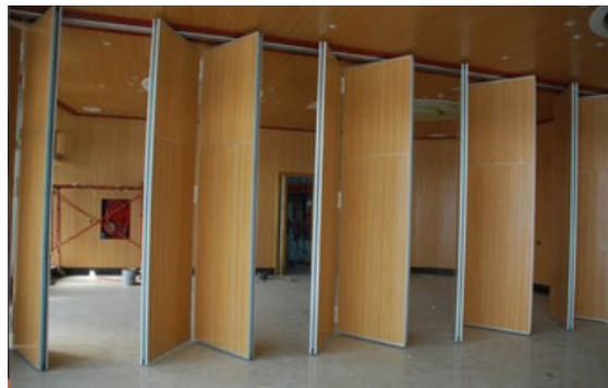
Fig. 15. Partition of the floor to small shops using light weight to help solve the problem of street vendors.
