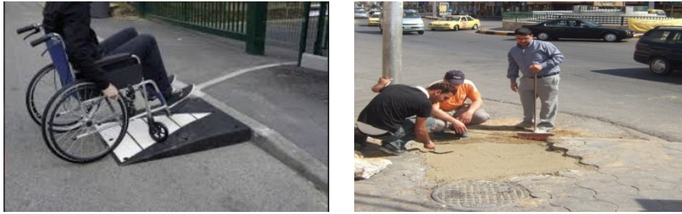
Figure 16. Add an earlier ramp to the pavement (on the left) and adjust the slope of the pavement after its collapse (on the right).
