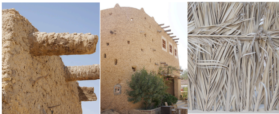
Figure 17: Use of date palm trunks as floor beams; Modern karshif building (Siwa Documentation Center of Cultural Heritage and Natural (; Fence made of date palm fronds. Source: ©Hermann (FAO, 2016. Accessed October 15, 2017, www.fao.org/3/a-bp825e.pdf .)
