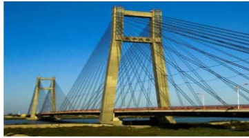
Figure 1 Photo of the Tianjin Yonghe Bridge
