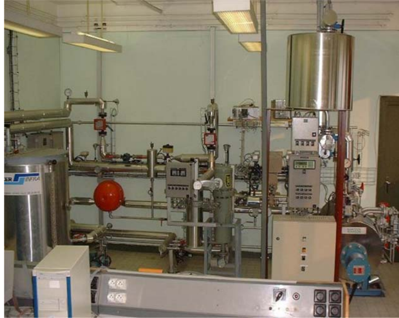
Figure 13. The steam generator installation
