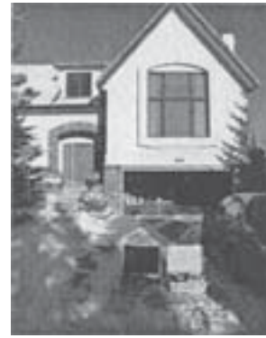
Fig. 1—Residential Garage Used for Test
