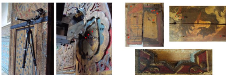
Figure 1. Photos of some zones of the carpentry studied in this work.
