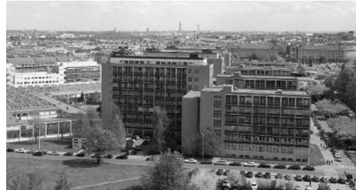
Fig. 1. The building of the Czech Technical University in Prague that was used for MPC application.
