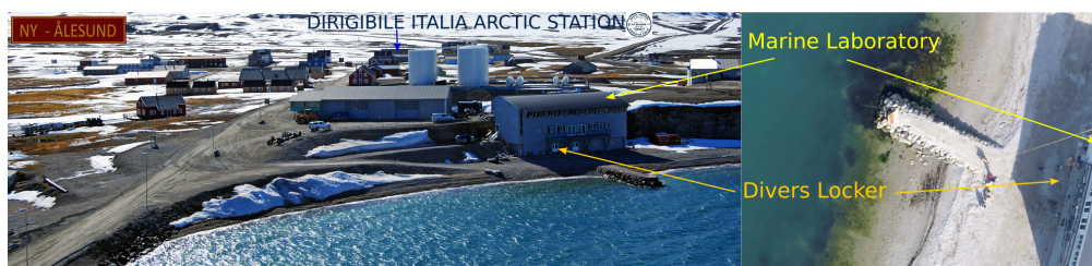
Figure 6. Ny-Ålesund and the infrastructures used by Italian National Research Council (CNR)-INstitute of Marine engineering (INM) researchers.
