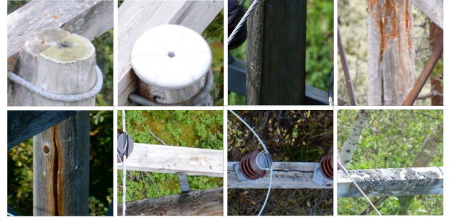
FIGURE 3. Sample images of the DS2_Tc, DS3_Po, and DS4_Cr datasets (from left to right, top to bottom): missing top cap, normal top cap, normal pole, woodpecker-damaged pole, cracked pole, normal cross arm, cracked cross arm, and rot-damaged cross arm.
