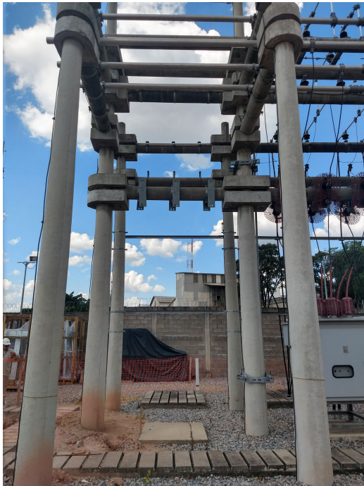
FIGURE 5. Free span, having built only the base.
