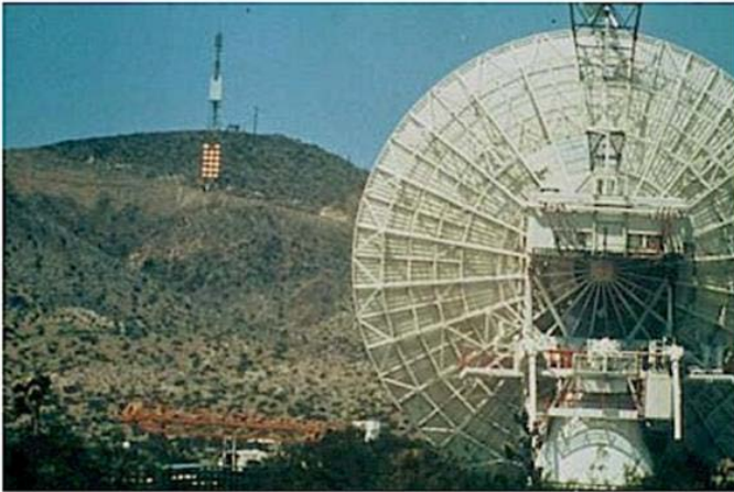
Figure 1.1.5: Venus Site of the JPL Goldstone Facility in California © [2018] IEEE [17]. The dish is used to transmit and the rectenna array is a panel seen in the distance.
