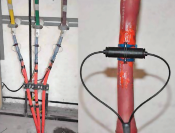
Fig. 2. Example of optical sensor fitting
