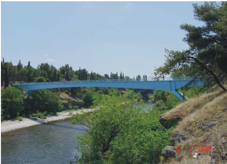
Figure 1: Photograph of the Podgorica footbridge.
