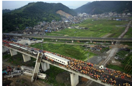
Figure 7. Derailment accident happened in Wenzhou, China
